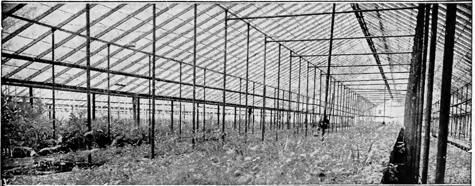
Interior photograph of our mammoth Rose-Growing Glass House, 300 feet long, 150 feet wide. Insect proof. Built of glass, concrete and steel. Will house one million young rose plants.
